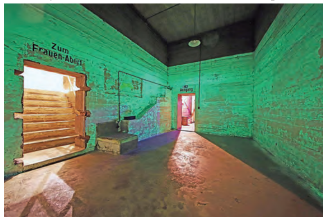
Worn but still effective, the luminous paint in the Gesundbrunnen bunker. Photo Berliner Unterwelten
